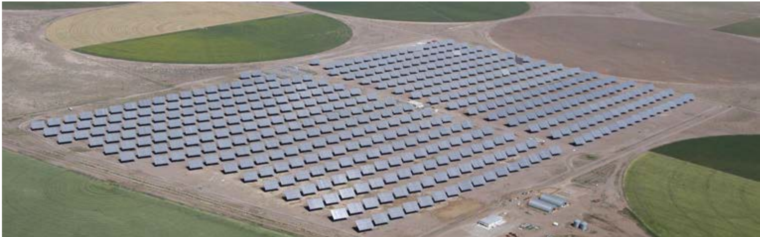
30 MW plant in Alamosa, Colorado, USA (© Amonix)
