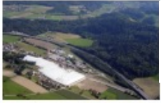
Hazardous waste landfill in Kölliken (AG)
