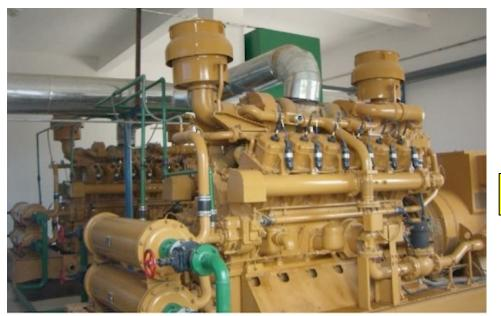
500 kW<sub>el</sub> biogas engine
