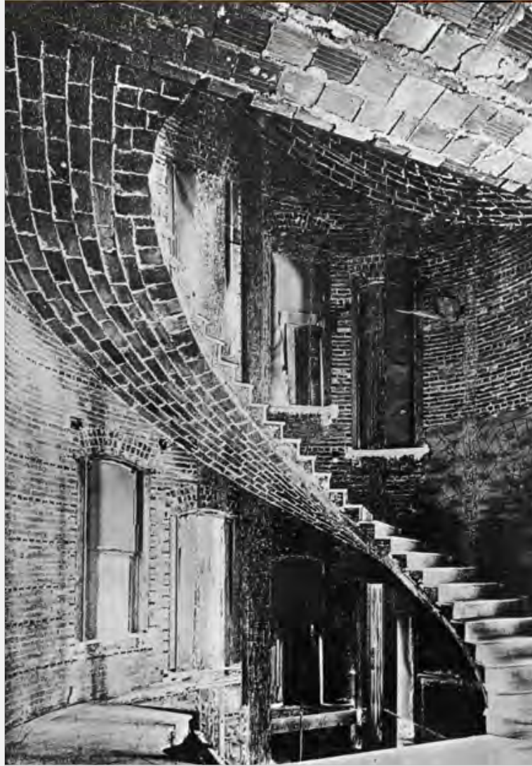
First National Bank – Guastavino 1890
