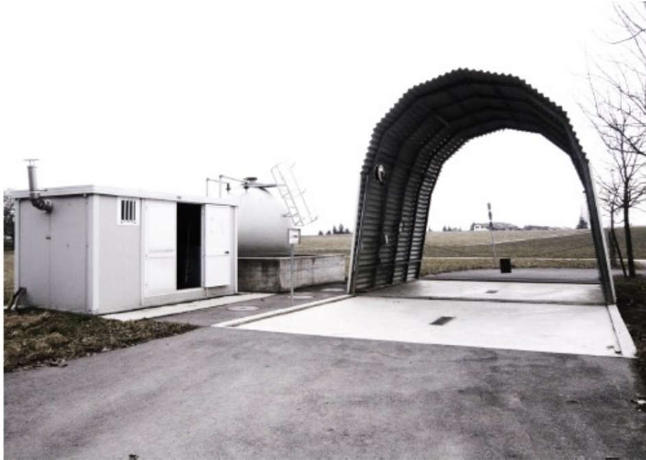
Washing station for agricultural equipment in Denens (pesticide contamination management)
